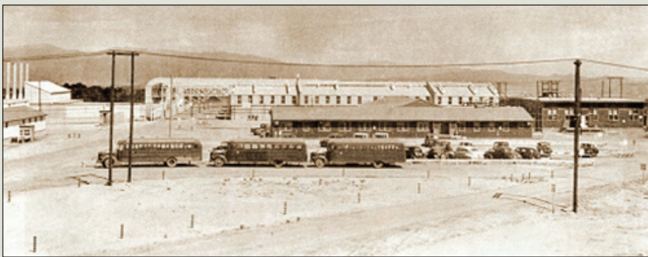
Plutonium operations moved to DP Site in 1945.
